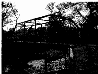
Lambs Creek Bridge, Jefferson Township
