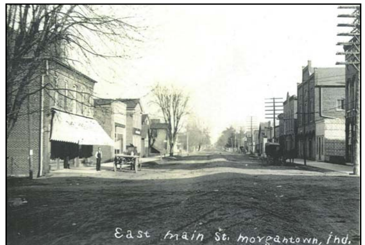
East Main St. (W. Washington St.) from Marion St. looking east, prior to 1908
